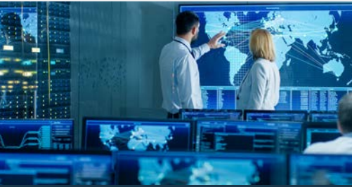
CONTROL ROOMS Video Wall Control & KVM
